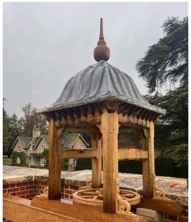
Bellcote after Restoration
